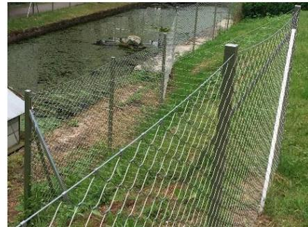
Guide the tensioning ropes through the middle posts at the top and the bottom. At one side insert the ropes into the rope tensioner
