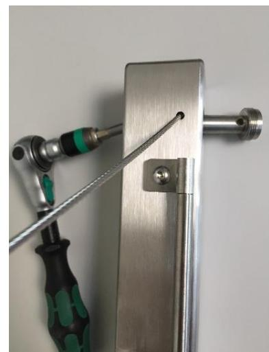
Turn the rope tensioner with a ratchet wrench and fix the rope tensioner with M3 screw at one of the four thread positions. Then cut the rope ends on the other fence side to the appropriate length (approx. 15cm longer than the end of the post). After that insert the rope into the tensioner and bring it to the desired or required final tension. Fix it again with M3 screw.
